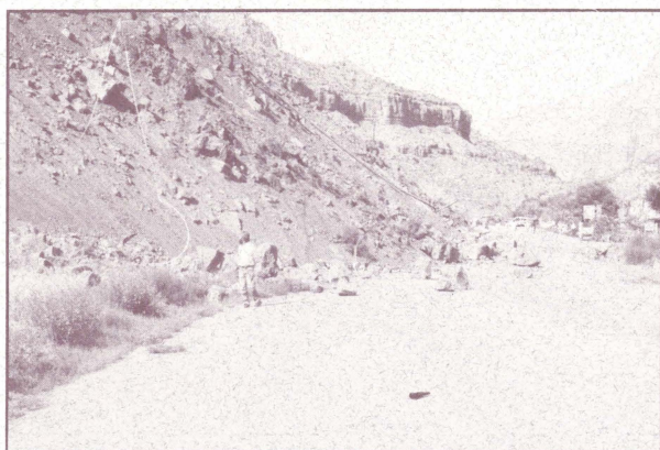
Figure 3. Toe of the Balanced Rock Hills landslide near State Route 9. Note ruptured utility lines in the toe of the slide. Photo by B.D. Black.
