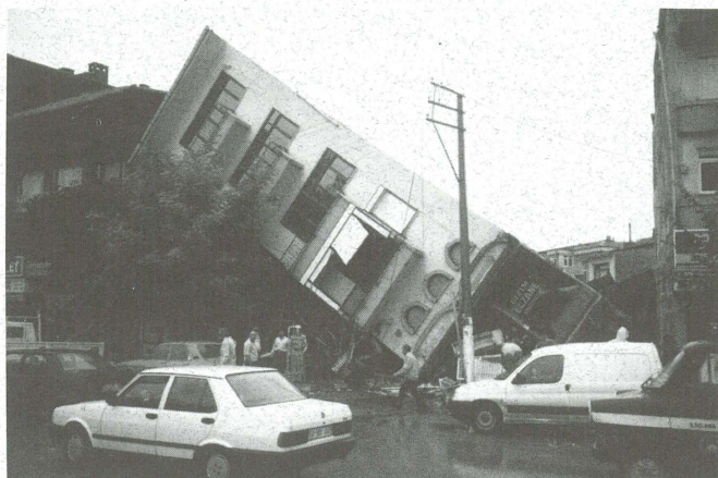
Although the structural integrity of some of the buildings was sound, liquefaction toppled them anyway
