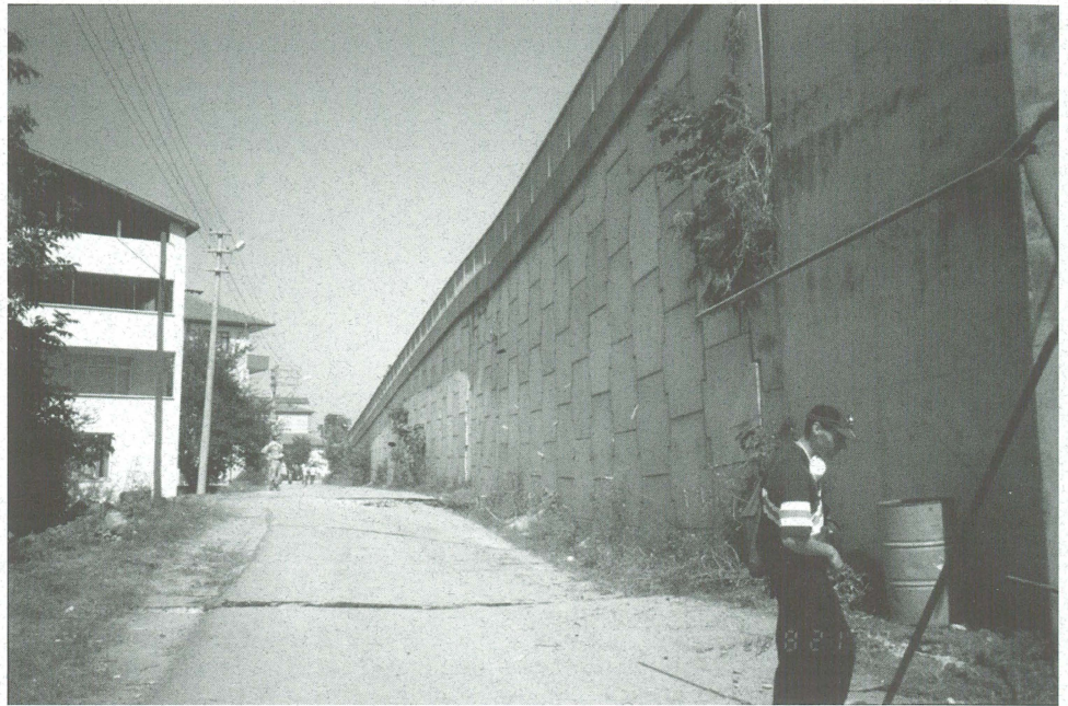
This mechanically stabilized earth wall, supporting a roadway, was within few meters of the primary fault rupture. Although subjected to differential settlement, it suffered only minor damage.
