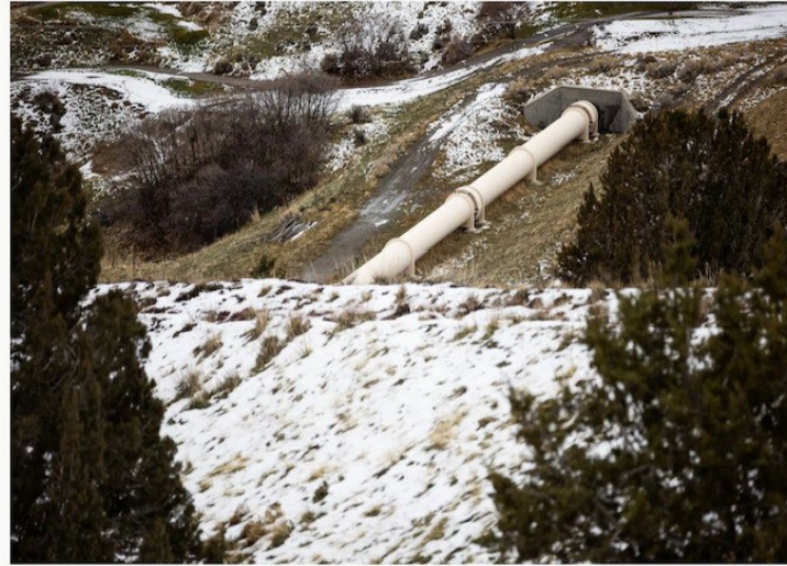
A section of the Alpine Aqueduct runs above ground where it crosses a fault in the hills above Orem on Thursday, Jan. 6, 2022. | Spenser Heaps, Deseret News | Purchase Photo
