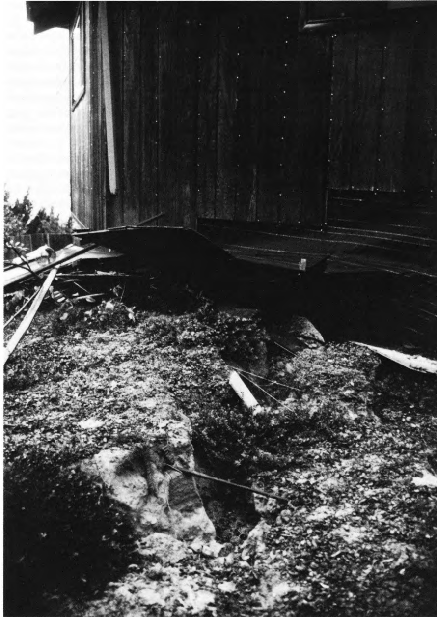
Figure 22. Scarps and cracks associated with movement of deep-seated slumps. A , Scarp at head of block slide in residential area of Brookdale in Santa Cruz Mountains. Block slide moved approximately 1.5 feet downslope (to right). Part of house to left of scarp remained on undisturbed ground while part to right moved downslope on slide block. Notebook on scarp is 8×10.5 inches. B , Home destroyed by landslide movement. Note cracks, from internal fissuring of landslide block, in pavement. Part of house on right has separated from part on left and tilted downslope as a result of differential movement within landslide block.
