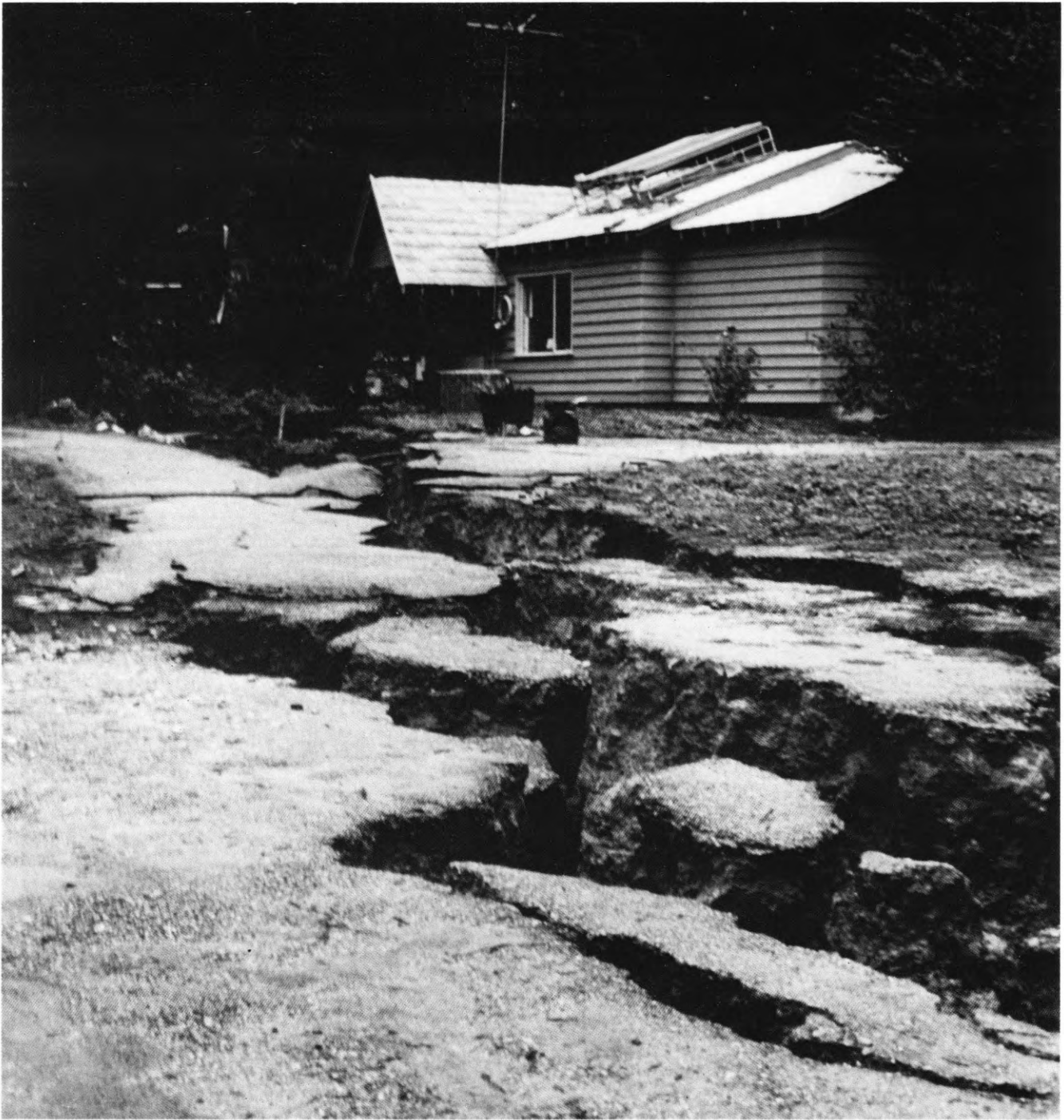
Figure 10. Crack system near Summit Road, 1/2 mile southeast of Highway 17. A , View northwest of wide zone of dominantly extensional cracks passing several feet in front of house. B , View southeast back toward house showing driveway dropped down relative to garage. C , Same crack where it crosses Summit Road; crack trends nearly north here rather than northwest and displays large component of left-lateral displacement. In general, upthrown block is on downhill side of this crack. Swale along crack on northeast side of Summit Road ridge in this area suggests similar displacement may have occurred in the past.
