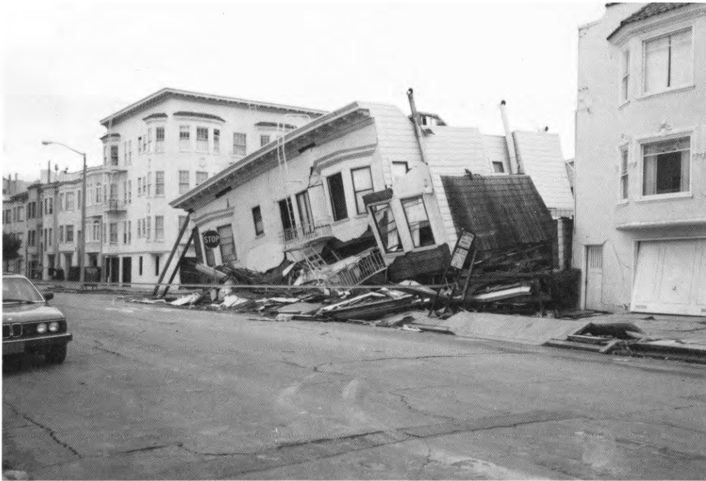
Figure 24. Structures damaged in Marina district. A , Damage due to ground failure of liquefied land fill. B , First story of this three-story building in Marina district was damaged because of liquefaction; second story collapsed. What is seen is third story.
