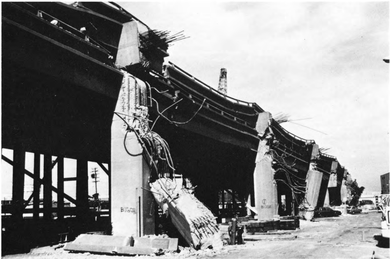
Figure 30. Collapsed Cypress structure on Interstate 880. A , Second deck collapsed onto first deck. B , Closeup of failed column that supported second deck. Only four 2-in.-diameter, steel reinforcing bars were used in this joint (foreground).
