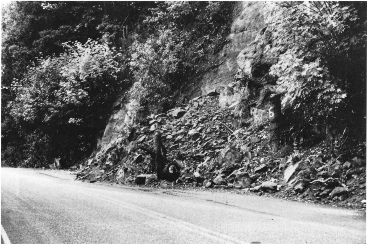
Figure 21. Small rock-fall deposit at roadcut, typical of those caused throughout Santa Cruz Mountains by Loma Prieta earthquake.
