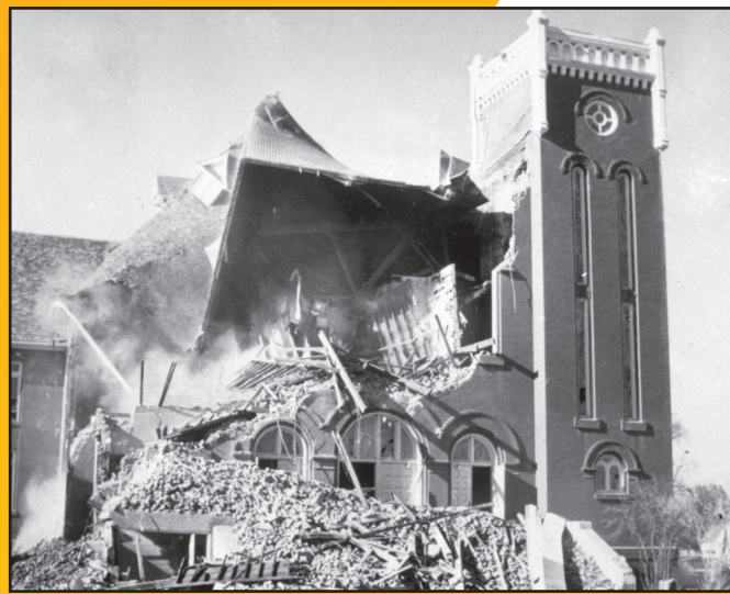
Benson Stake Tabernacle being demolished due to damage from the 1962 magnitude 5.8 Richmond earthquake in Cache Valley, Utah. Photo courtesy of the Utah Geological Survey.
