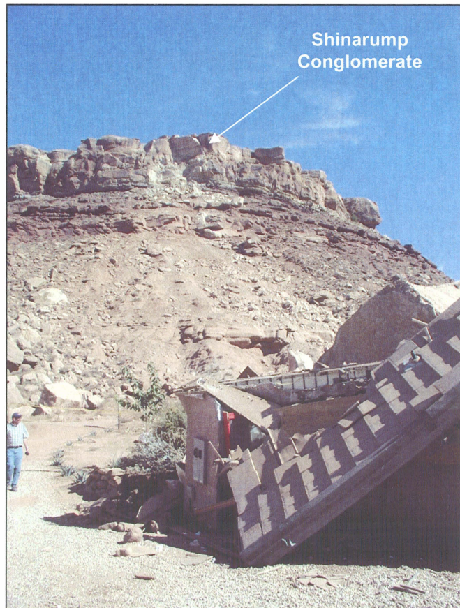
Figure 18. Shinarump Conglomerate overlying the upper red member of the Moenkopi Formation above the damaged home. Note the fresh scar where the rock fall detached from the cliff.
