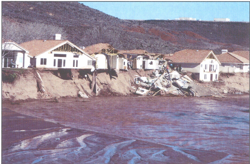
Figure 4. Damage to homes caused by flooding in January 2005.
