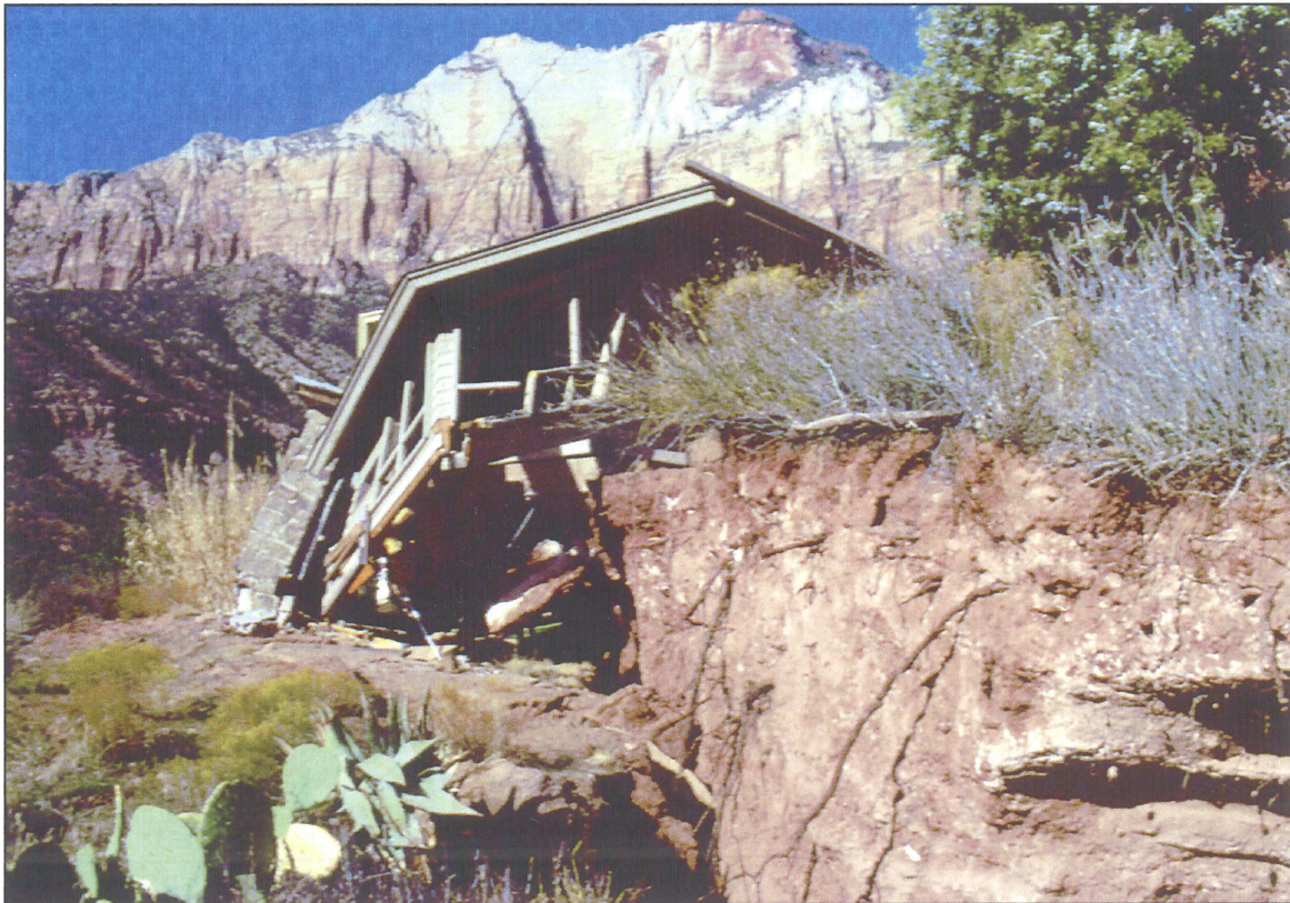
Springdale landslide in Springdale, Utah, which moved in response to the 1992 M 5.8 St. George earthquake.
