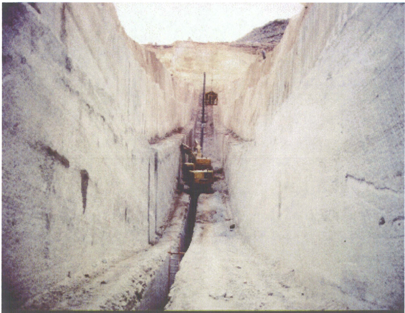
Figure 8. The Quail Creek south dam cutoff trench during reconstruction.
