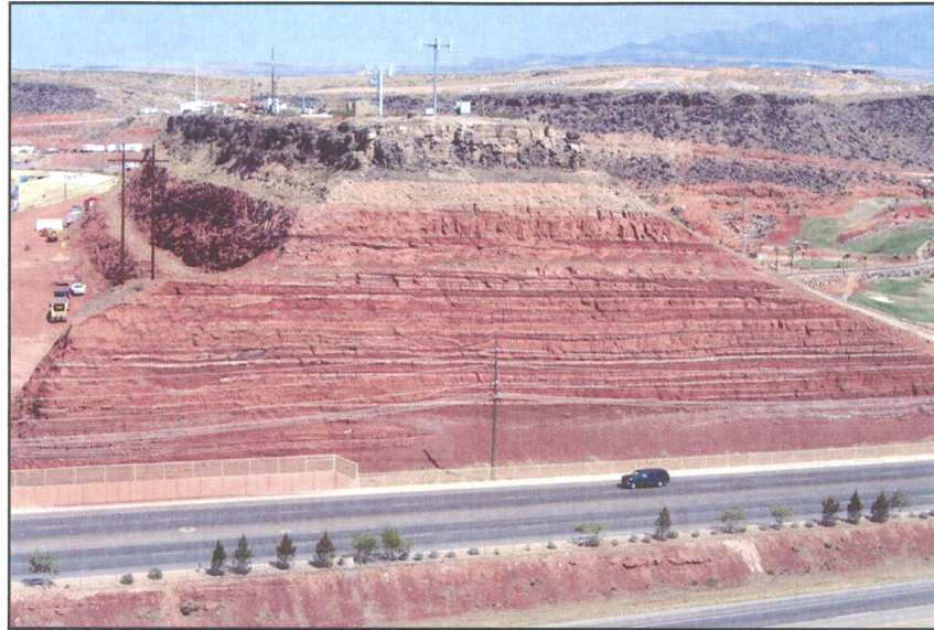
Figure 3. Road cut on the southbound side of I-15 through Middleton Black Ridge. Early Jurassic Kayenta Formation is capped by Quaternary fluvial deposits (light brown outcrops), which are in turn overlain by a Pleistocene (1.5 Ma) basalt flow (black) that originally flowed down the channel of a tributary of the Virgin River (photo courtesy J. D. Harris, Dixie State College).
