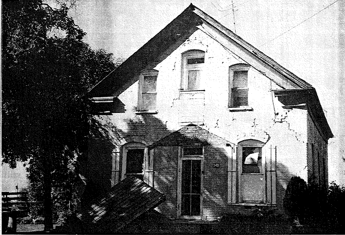
Figure 2: Cracks/failure due to earthquake
