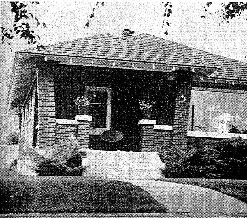
Figure 10: Another URM pier failure.
