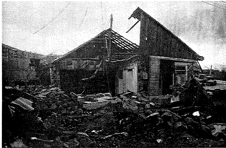
Figure 3: Unreinforced masonry collapse
